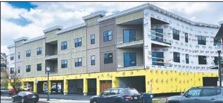
The Point at Broad Street — Developer Chris Patten's project at the former Rite Aid site on South & Broad Streets. Exterior finishes are underway, the ground floor parking lot is in use.
