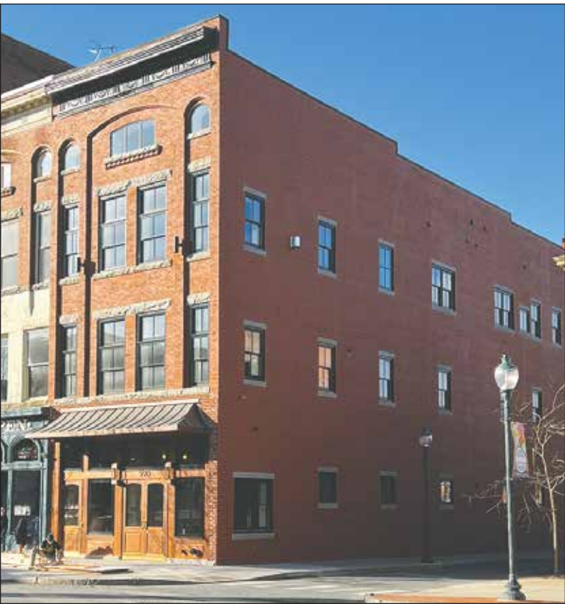
Before: The solid brick north wall. Now: Windows on all three floors — and light flowing into the building.
